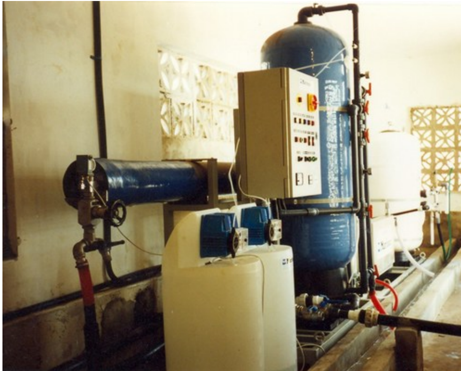
Installation of WDS in Lampedusa Island Resort (Italy)
